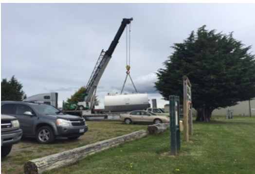
Installing above ground aircraft fuel tank
